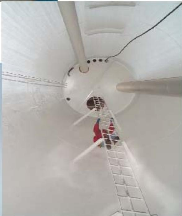
← That is Brandon hanging out of the access port rigging the pulley for the ground crew to hoist the coax, antenna and tool bags up.
